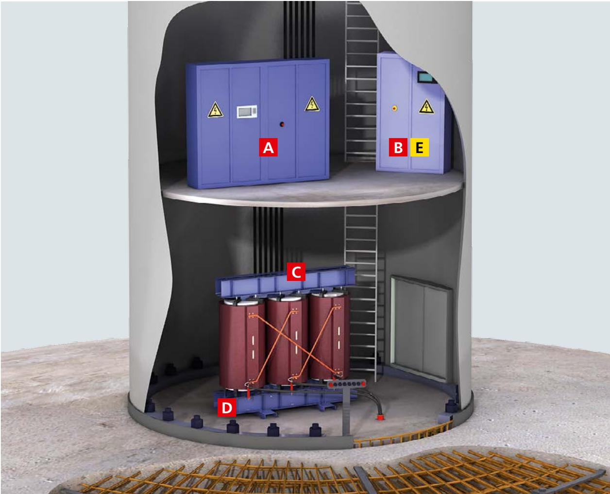
A comprehensive lightning protection concept comprises the protection of the nacelle and surge protection in the tower base. In the tower base, both the medium- and low-voltage power side and the data side require protection.
